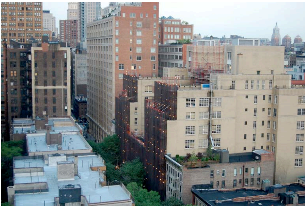
Illuminated scaffolding of Fashion High at dusk.
