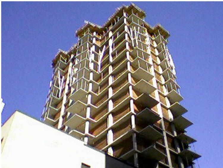
One block north, at 52nd Street, just east of Second, nineteen floorsworth of what was to be a 46-story condo, and from whose face – in the gap between the two rows of terraces on the right – the crane sheared away. Resembling pediments, the wooden forms built to receive the next floor's concrete pourings remain, whether expectant or resigned to decay, hard to tell from any photo. This may be the largest single pigeon coop in Turtle Bay, and perhaps even in the whole of this great city. For now.
